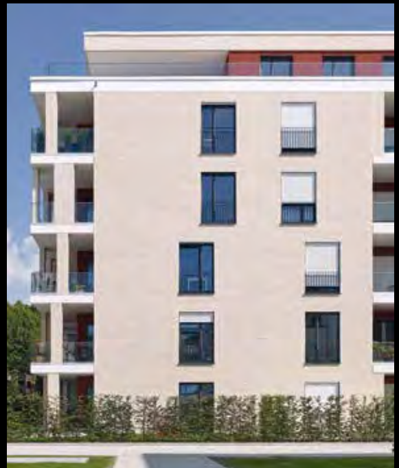
Private home, Cologne, Germany clinker brick slips 7470/351 kalkbrand corner 7471/351 kalkbrand
