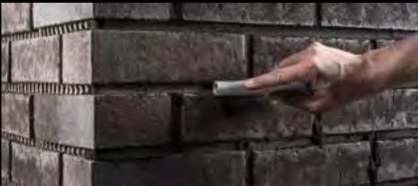
Jointing with a trowel allows you to create different looks.
