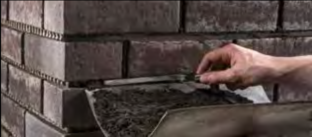
Grouting using pointing trowel and metal float along the horizontal.
