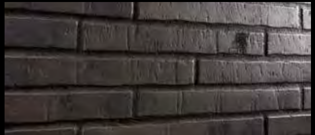
The finished joint pattern after slurry treatment. A wall surface from the GLANZSTÜCKE series.
