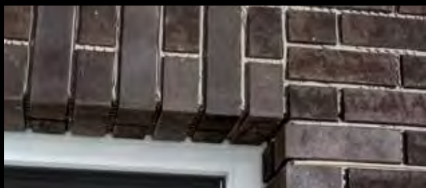
Window lintel perfectly replicated with angles.
