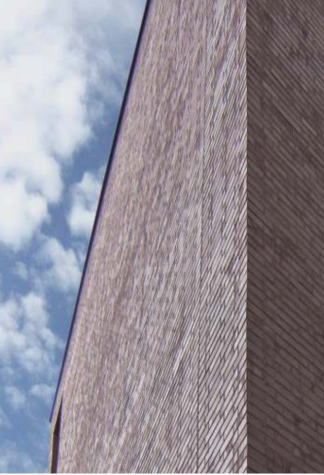
1828/0 Aubergine smooth, corners manufactured to specified angle, Project: KerVita Hamburg
